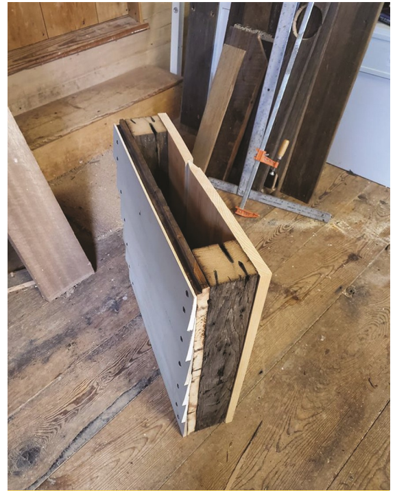
Cross section of external wall with spruce siding on the outside and paneling on the inside. This will be shot at with replica muskets to visualize the results and also be used as a hands-on component in the new exhibition.
