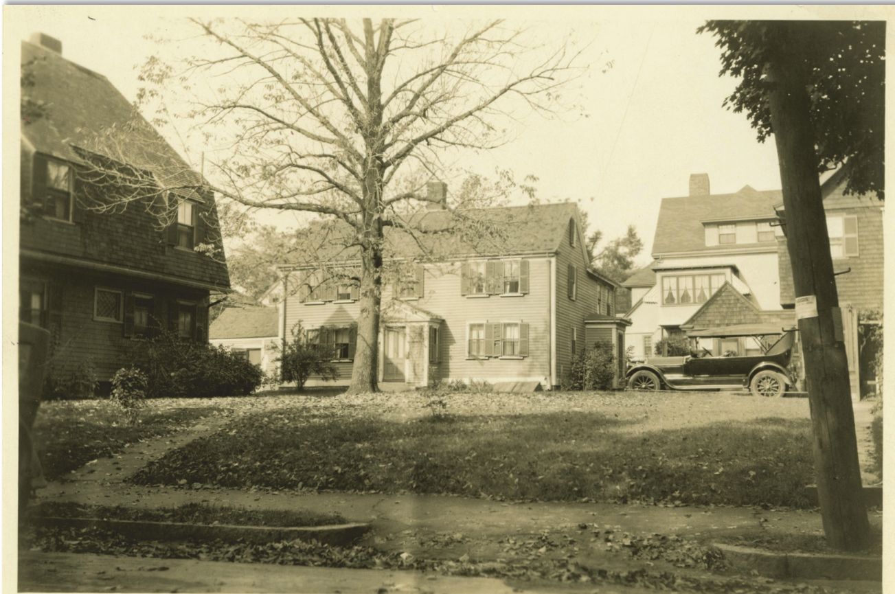
This 1922 photograph of the Jason Russell House. Hemmed-in by other buildings and occupying just a 60 x 80-foot lot (4,800 square feet), it was only accessible from a narrow pathway. The house shows signs of disrepair, such as the exterior window shutters, and had been modernized with Victorian-era two-over-two large-pane windows.
